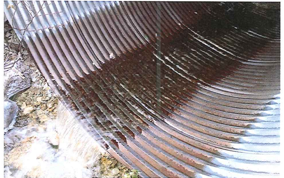
CK2208 Floor Rust
